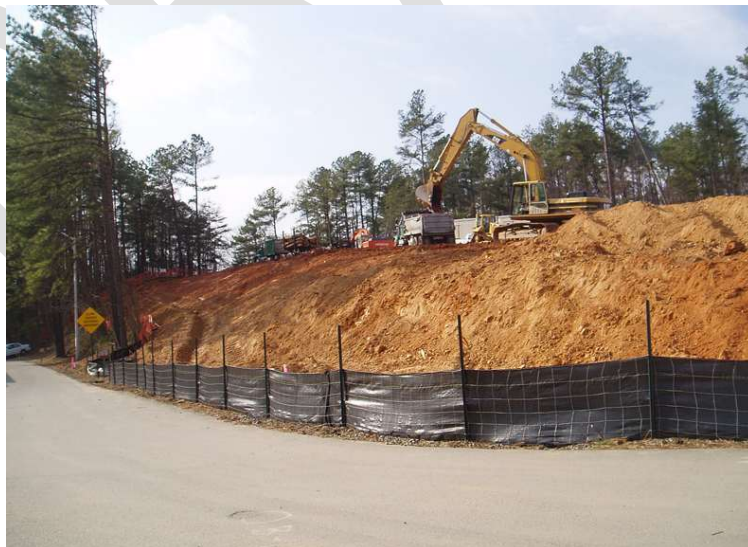
Silt Fence for Erosion Control
