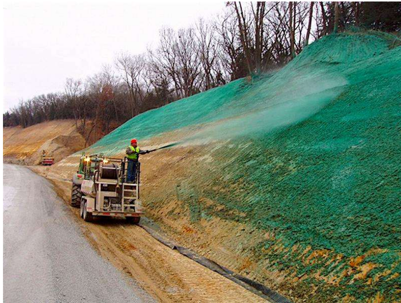
Hydroseeding for Erosion Control
